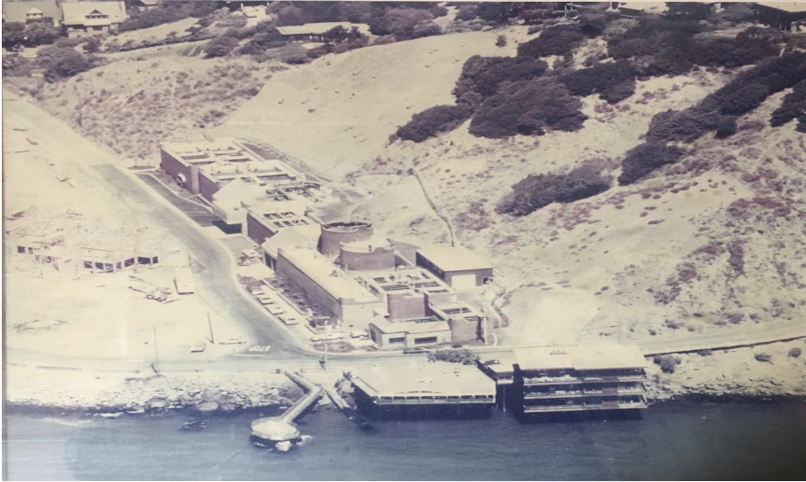
1980's era- Tiburon Peninsula- Secondary Treatment additions to Wastewater Treatment Plant
