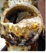
Disposing of fats, oil and grease down the drain can quickly lead to clogs like this! Do your part to keep it out of the sewers.
