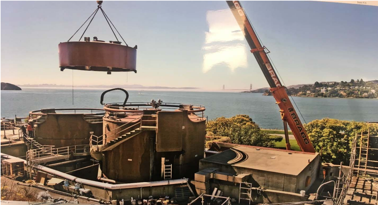
2014 – Tiburon Peninsula –Main Plant Rehabilitation at Wastewater Treatment Plant
