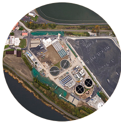
City of Everett | Collection System Odor Control Plan Everett, WA
