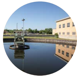
Johnson County Wastewater | System-Wide Integrated Plan, CIP Prioritization, and Asset Management | Olathe, KS
