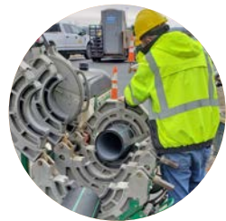
City of Winston-Salem | Collection System Improvement Winston-Salem, NC
