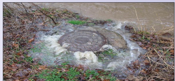
This photo of a sewer system overflow was not taken in our District.
